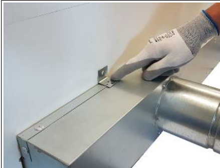
Fig. 4: Positioning the brackets
