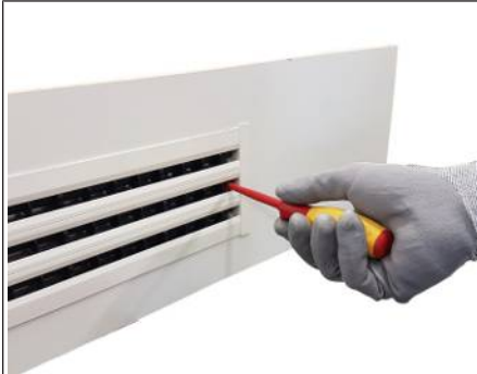
Fig. 11: Loosen screws on the left and right.
